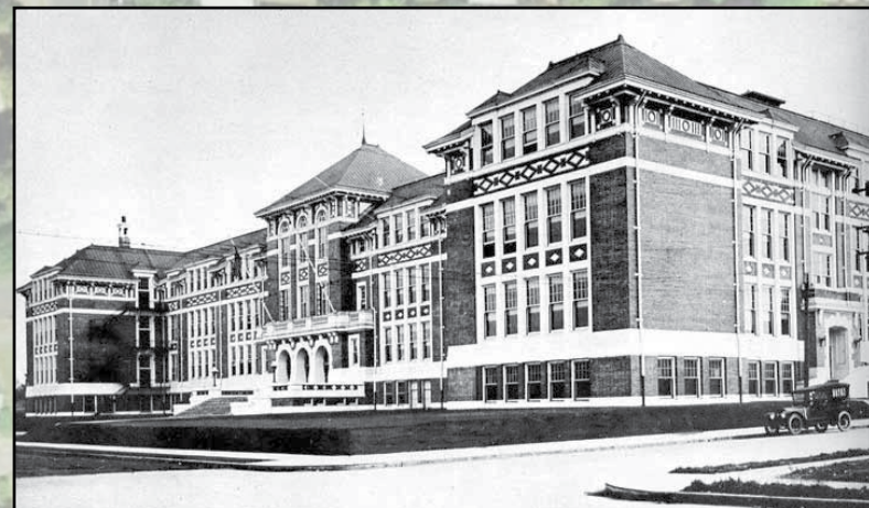
1910s photograph of Jefferson High School, looking east.
