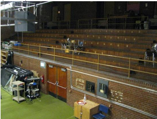
View of old (1928) gymnasium seating
