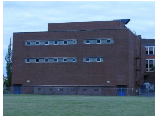
South elevation of 1952 auditorium addition
