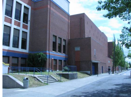
View of 1952 auditorium addition, looking south.
